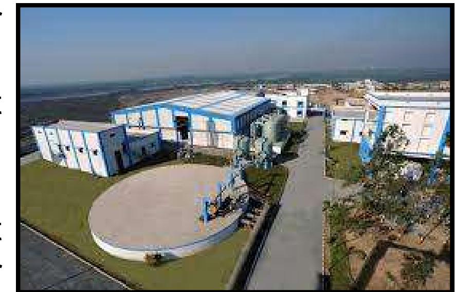
Bamroli Sewage Treatment Plant
